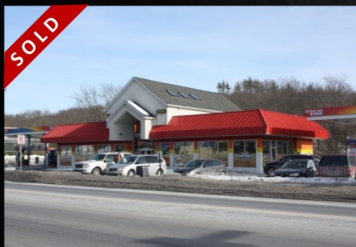
Sunoco Gas Station
